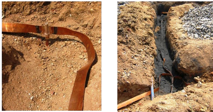
Figure 3.4 : Interlinking of earth pits using copper tapes
